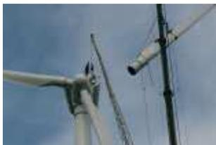
The nacelle, which typically contains the gear box, low- and high-speed shafts, and the generator was lifted and set on top of the tower.
