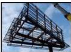
A new tri-face head, engineered for one of the 20' x 60' faces to be digital, and the option of upgrading the 20' x 36' face to digital was assembled and flown.
