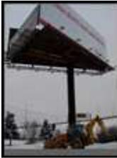
This month's project was the upgrade of a structure to digital capable. The existing structure was a tri-face; two faces 20' x 60' and one face 20' x 36'.
