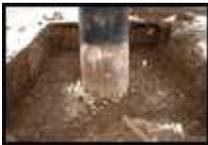
First, we had to modify the foundation; excavating 3 feet below grade and adding rebar.
