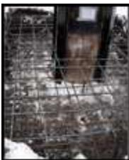
Structural beams could then be welded to the column extending into the excavated area. A bonding agent was added and concrete poured.
